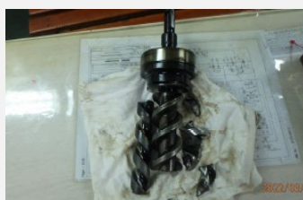
DAMAGE TO FUEL CIRCULATING PUMP
